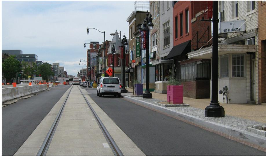
One-half of constructed roadway, which includes two travel lanes - one shared with streetcars, a designated parking lane, and a sidewalk area.
